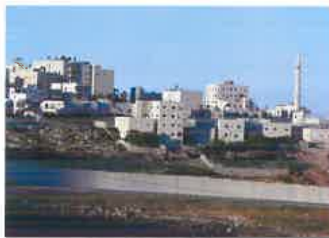
▲ FIGURE 6-65 SEPARATION BARRIER The minaret tower of a mosque in East Jerusalem can be seen in the image.
