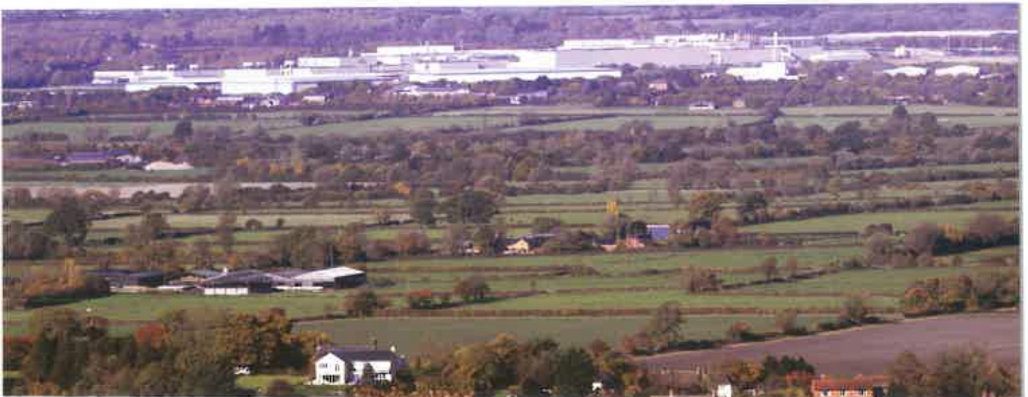
▼ FIGURE 11-26 MODERN ONE-STORY FACTORY The Honda assembly plant in Swindon, United Kingdom, is spread out over one story.
