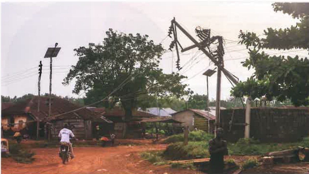
◀ FIGURE 11-55 SOLAR ENERGY Solar panels generate electricity in Odoru, Nigeria.
